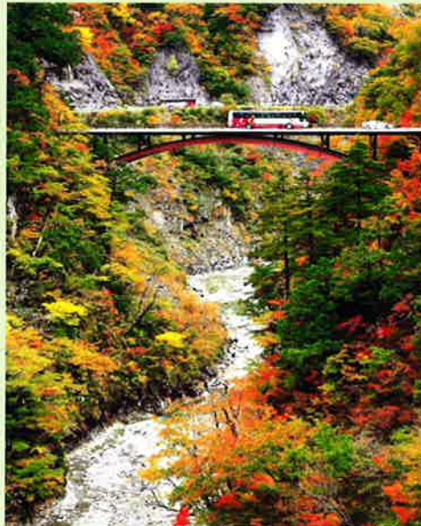
Jatani Ohashi Bridge in autumn
